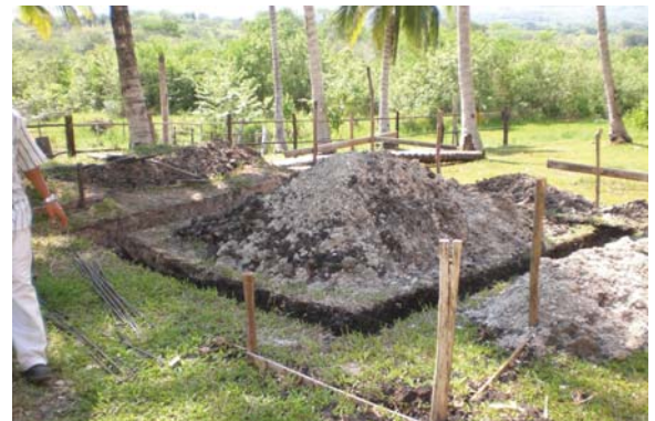
Layout complete and foundation trenches excavated.
