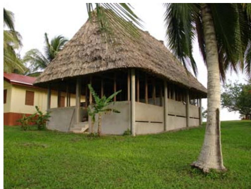
North facing end of Bird Rehabilitation building. Additional progress photographs on page 3.
